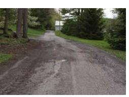
Before paving, a roadway must be prepared through proper pothole repairs, base repair, crack sealing, or scratch and leveling courses to address surface irregularities and provide a uniform foundation. Photo: PennDOT LTAP
