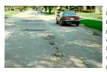
Before paving, a roadway must be prepared through proper pothole repairs, base repair, crack sealing, or scratch and leveling courses to address surface irregularities and provide a uniform foundation.
