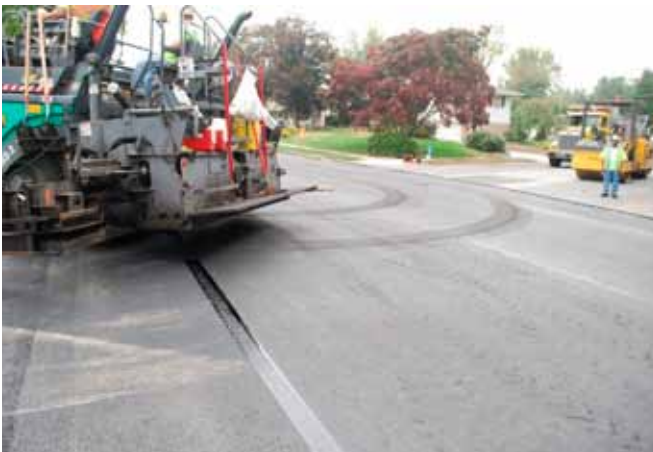
The paver turns on the paving fabric without damaging the fabric. Loader tri-axle trucks also traveled across the fabric with no resulting damage. Photo courtesy of ISMF LLC.
