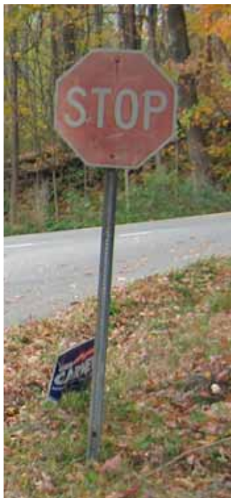
The intent of the standard is to identify and replace signs that no longer meet the needs of nighttime drivers.
