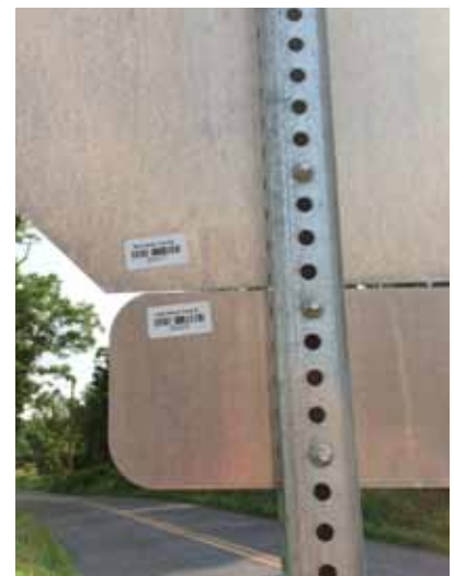
One method for tracking sign inventory is to use a bar code.
