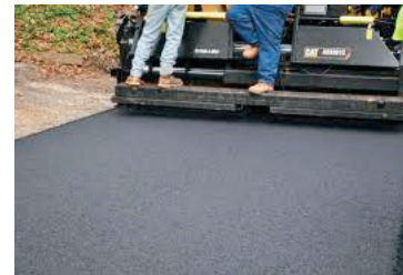
Road crews that use Warm-Mix Asphalt like how the mixture is produced and placed at lower temperatures.
