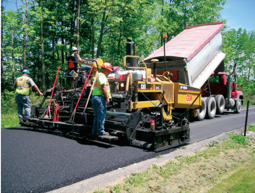
Warm-Mix Asphalt being applied on Route 2012 near Spring Mills, Centre County.
