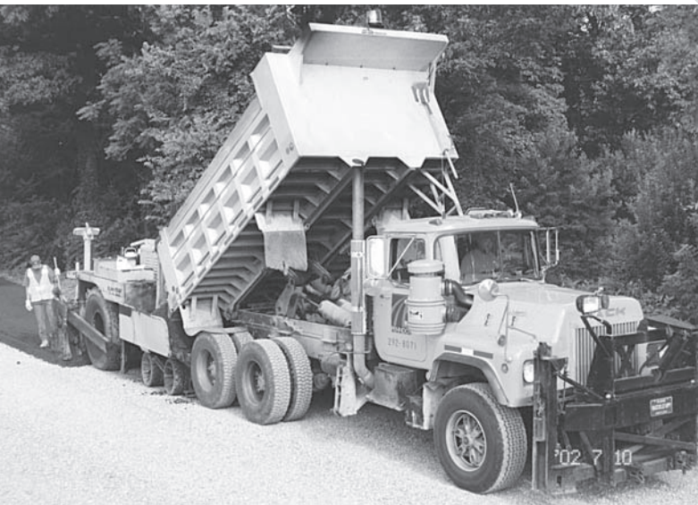
PennDOT placing millings on Gurtner Road through AGILITY program.
