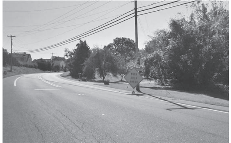
On local roads in non-urban areas, temporary traffic signs at work zones must now be spaced at 500 feet.
