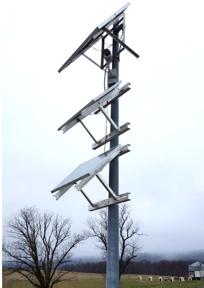
New Virtual WIM Camera and Solar Panels in Berks County
