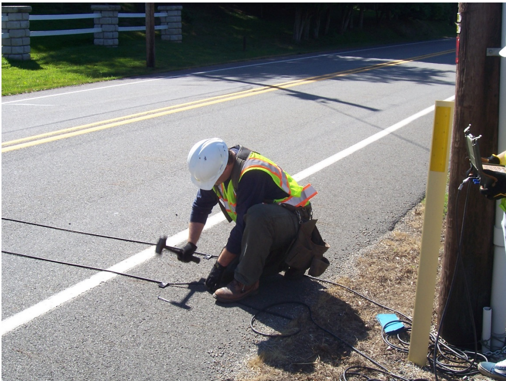
Short-Term traffic count being installed.
