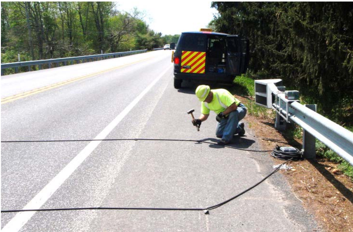
Short-Term traffic count being installed by PennDOT staff.
