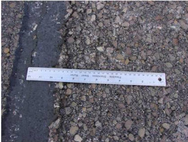
(b) high severity longitudinal crack along the left edge of the passing lane, 188m north
