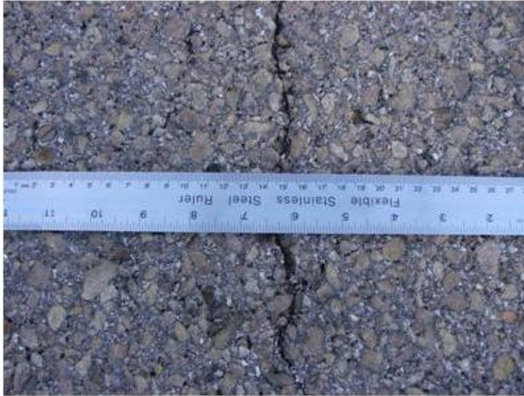
(a) low severity longitudinal crack along the right edge of the travel lane, 145m north
