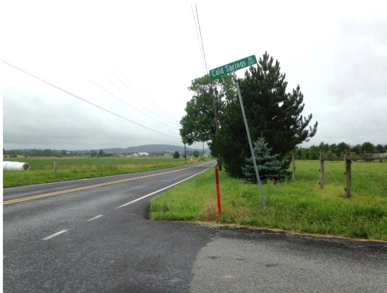
A solid-white line delineates the edge of a two-lane, two-way road. The line is broken at an intersection.
