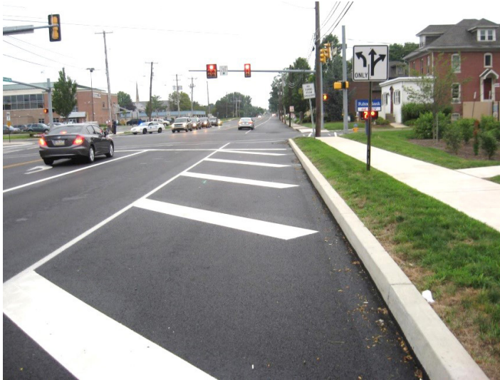
Edge lines and diagonal hatching can be used to help keep vehicles off a shoulder.
