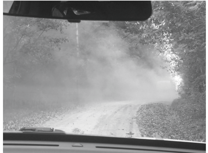
Dust indicates the road is deteriorating.
