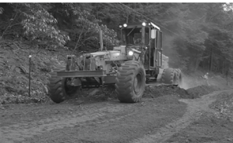
A grader is used to reshape the road surface of an unpaved or gravel road.
