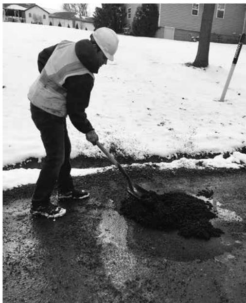
The success of your patches relates directly to how well you prepare holes and compact the patching mixture.
