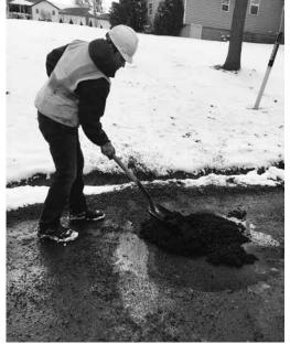
The success of your patches relates directly to how well you prepare holes and compact the patching mixture.
