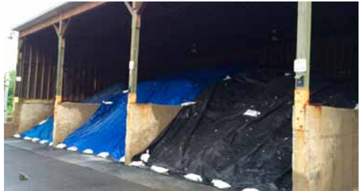
Make sure you cover or store your road salt under roof to prevent runoff and potential environmental contamination.
